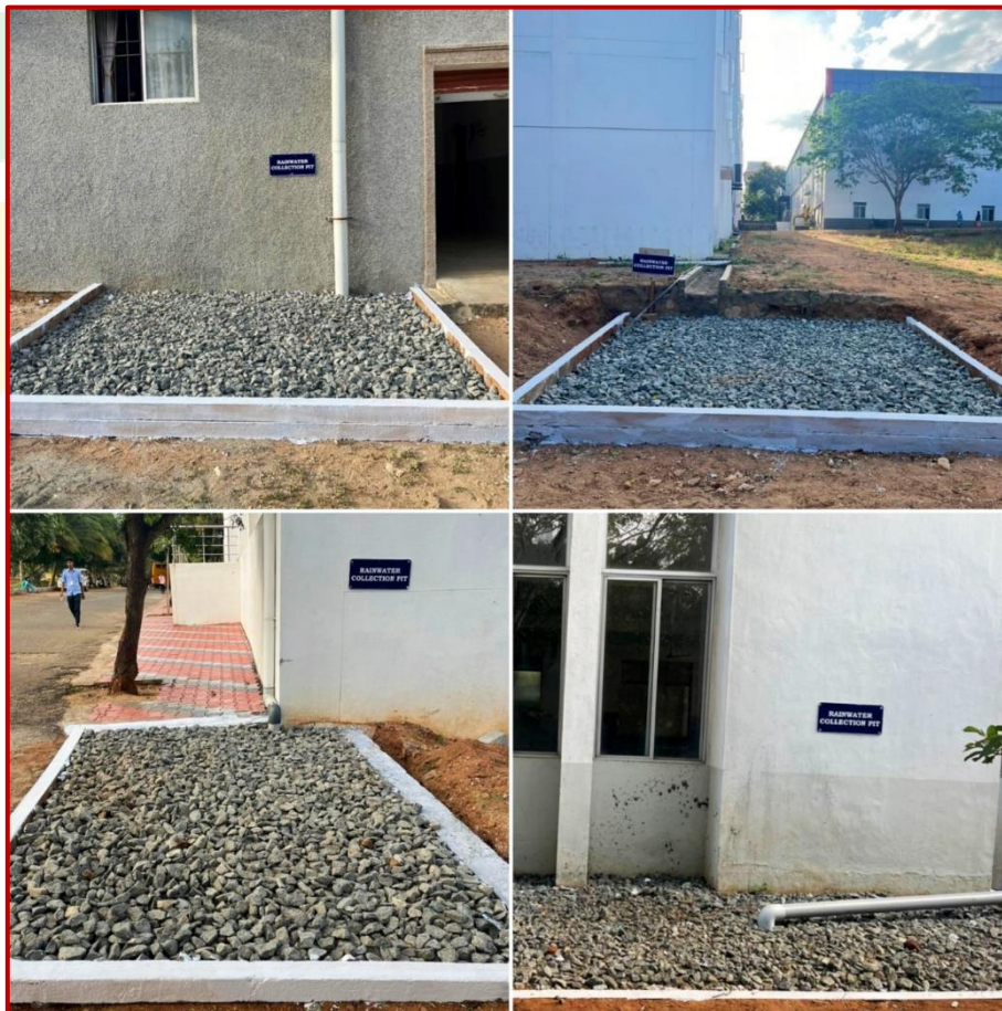
Rainwater Harvesting Pits
